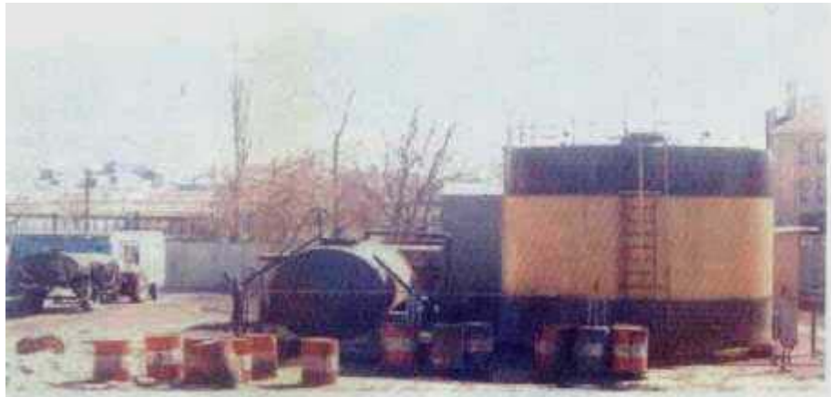
The bilge water collected from vessels is stored in the tanks shown in above photograph and segregated via settlement procedure (Haydarpaşa Port).
