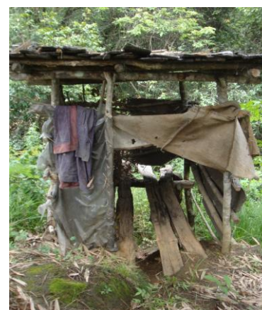
Hanging Toilet in Barilum, Kabjisa, Punakha.
