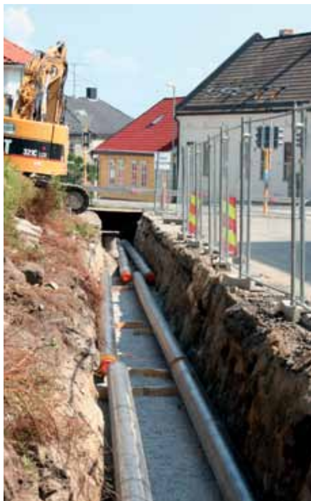
District heating development. Photo: Cathrina de Lange / Østfold Energi AS
