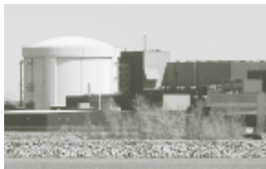
Gentilly-2 nuclear generating station.
