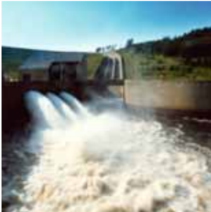
A 6 megawatt hydroelectric power station at Kielder Water, Northumberland.
