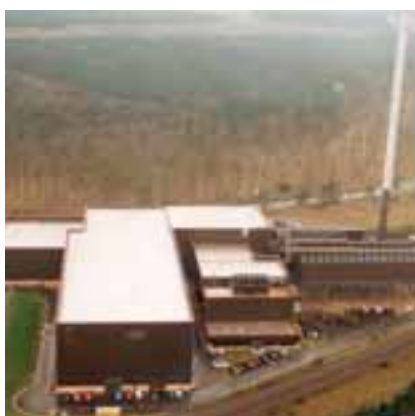
A chicken litter power station at Thetford, Cambridgeshire supported under NFFO 3.
