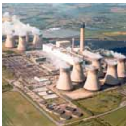
Drax Power Station, one of the largest power stations in the United Kingdom, co-fires biomass fuel with coal.
