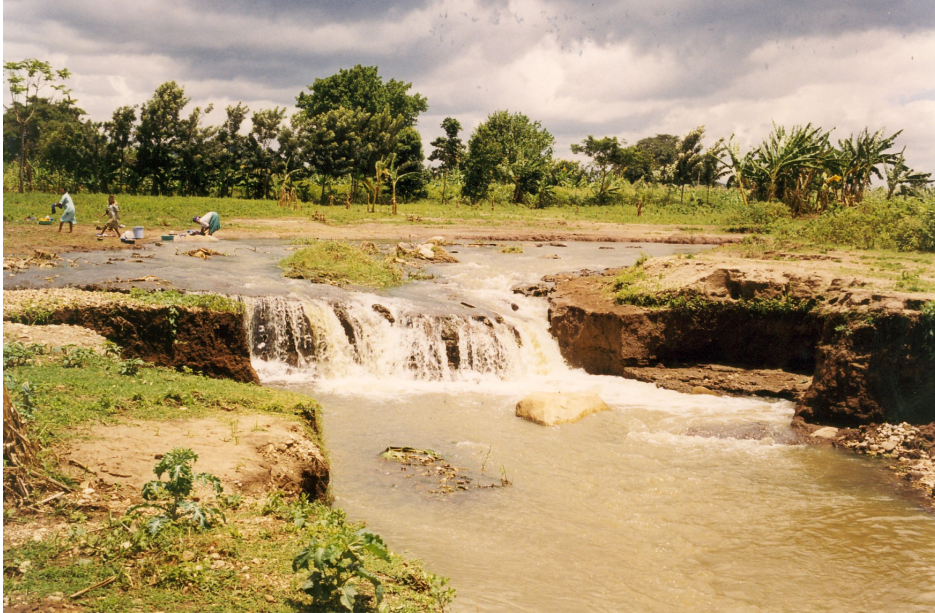
Figure 3: After the water had washed away the earth embankment, the water started creating a gully. The picture is taken upstream. The demolished embankment is behind the bush to the right in the picture.
