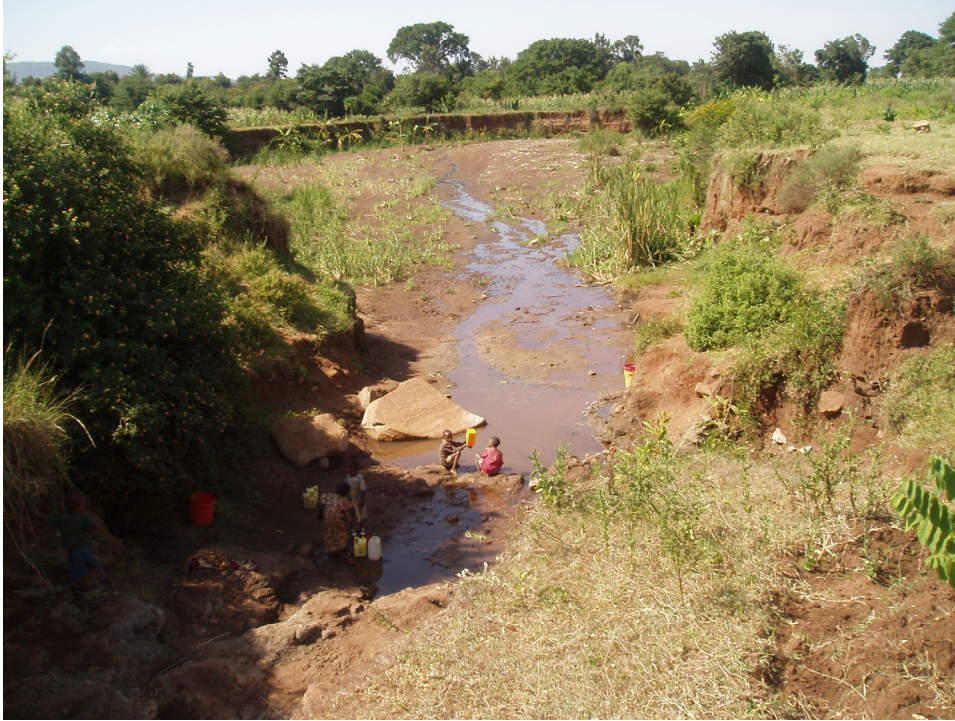
Figure 5: The same gully from the same vantage point as the previous picture. However, this picture was taken in February 2005, seven years later. The water has continued to erode and enlarge the gully considerably.
