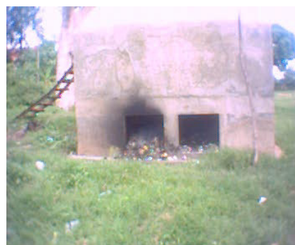
Fig.4: Incinerator as seen from behind un-burnt waste mixed with burnt waste ( Jinja Hospital )
