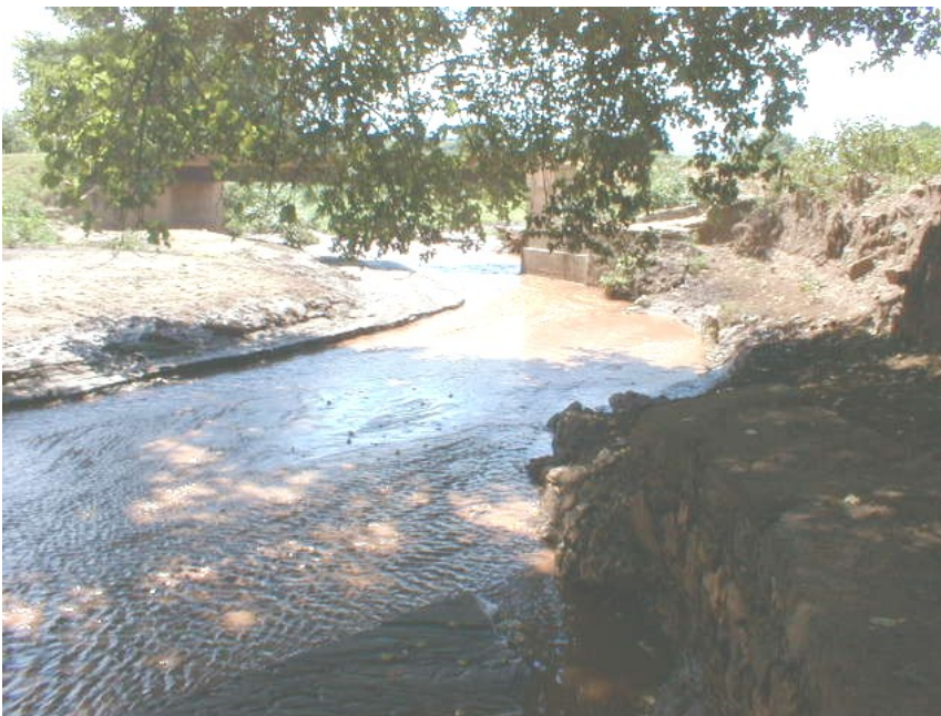
Figure 2: This picture, probably taken in 2004, shows that the original retaining wall is not there. The water has eroded the Arusha – Babati trunk road to the right of the right abutment of the Kiongozi Bridge.
