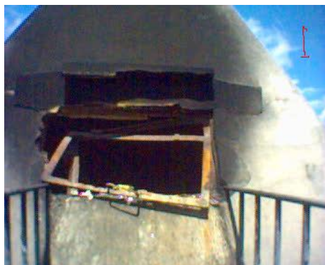
Fig.1: Opening to the incinerator (Masaka Hospital)
