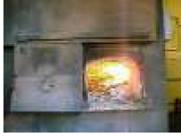
14 Incinerator ignited before being cleaned and cleared
