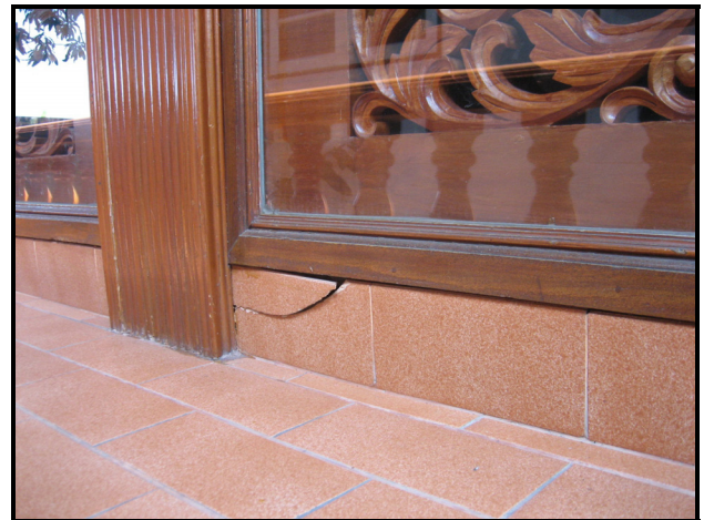
Impacts on cement walls due to the vibrations from take-offs and landings
