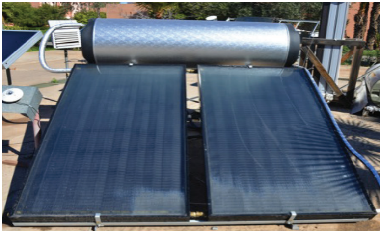
Figure 6 Solar Hot Water
