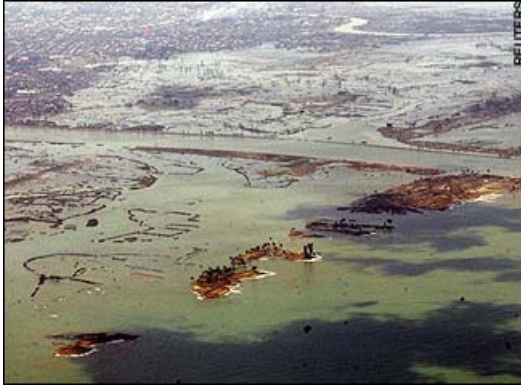
Exhibit 4. Damaged Coastal Areas
