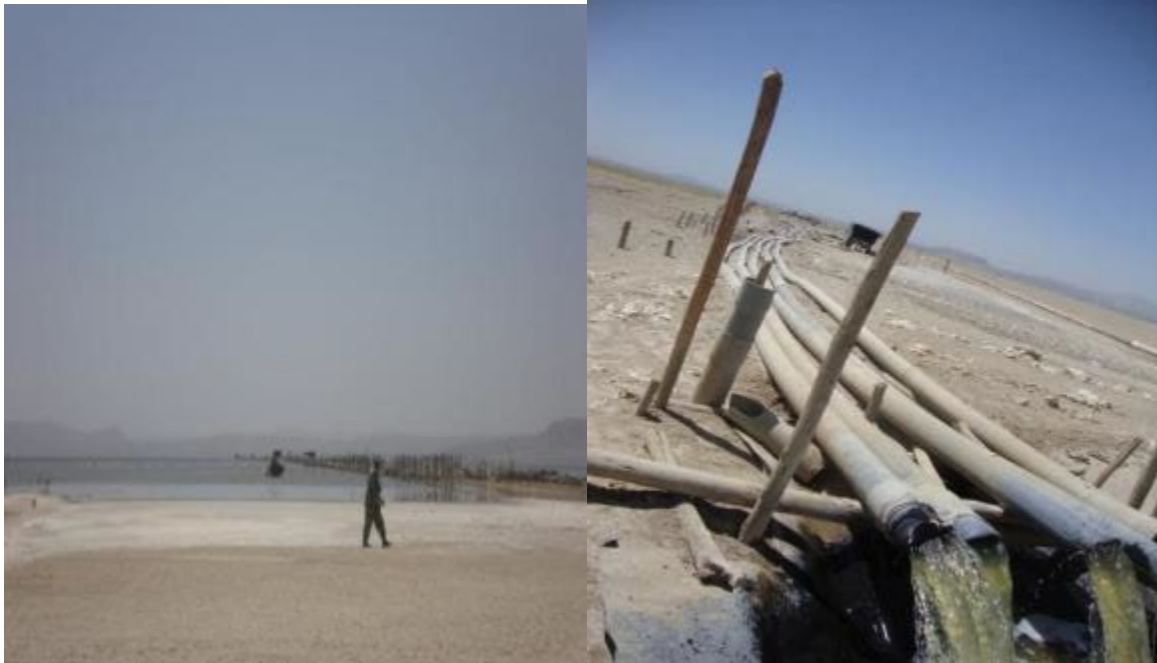
Water pumps and pipeline from Lake Abijata for Soda Ash factory
