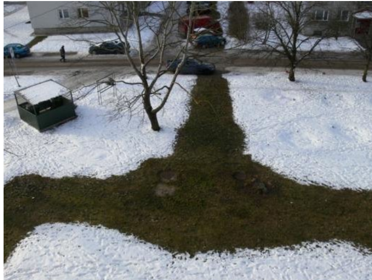
he pipeline heat loss is especially visible in the winter season. Source: toomas.trapido.org
