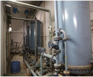
Sewage Treatment Plant (STP) of 40 Cu. M. per day for waste water treatment and reuse. Grey water is treated within campus and used for the gardens. Drip irrigation method is also used for water conservation
