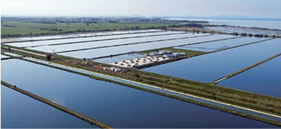
Excursion: Melbourne Water Werribee Treatment Plant and Ramsar Wetland
